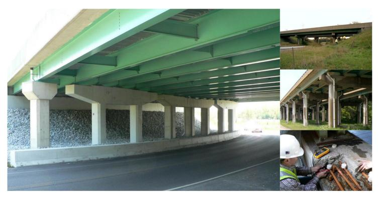
Within the Extension of Structures Project, an analysis has detected an important existing deterioration in the elements of the structures after 50 years of service, due to the salts in the freeze/thaw process.
